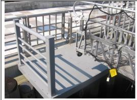
Design and/or park rules do not allow gangways to rest on the walkway of the pier, so permanently moored vessels are obliged to create a design that would have their gangway outboard of the fence. This cantilevered platform was designed and fabricated by ship LILAC.
