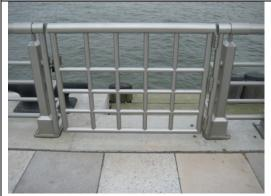
Gangway gate aligns with piling and cleat so gate cannot be used for gangway
