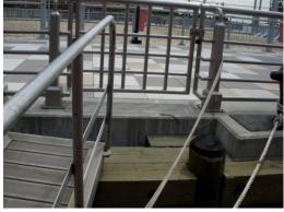
Gangway gate aligns with electrical grounding cord (at right under gate) so gangway cannot go there
